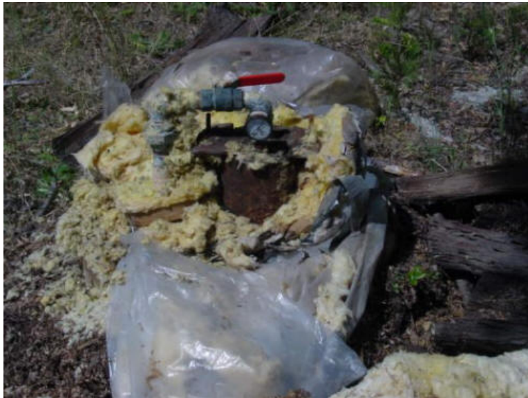
This is the main artesian well that fills the three tanks.
