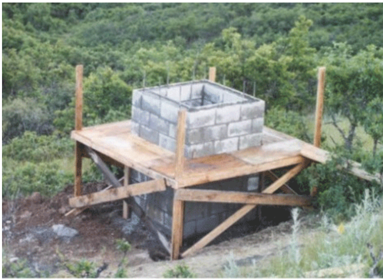
Value Beamer under construction.
