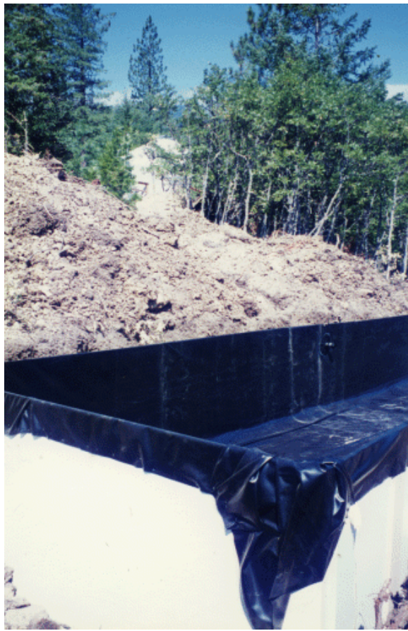
This is a septic tank. We built it big because we knew we were full of shit.
